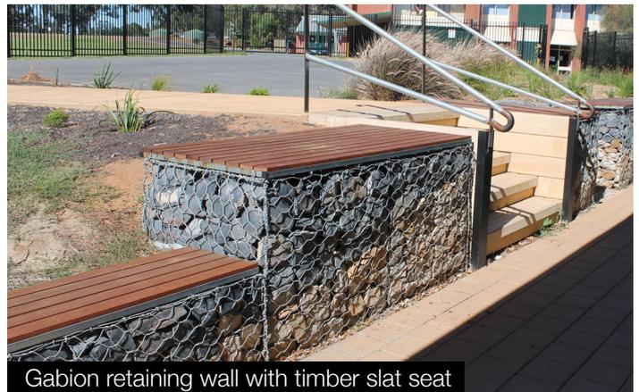
Gabion retaining wall with timber slat seat
