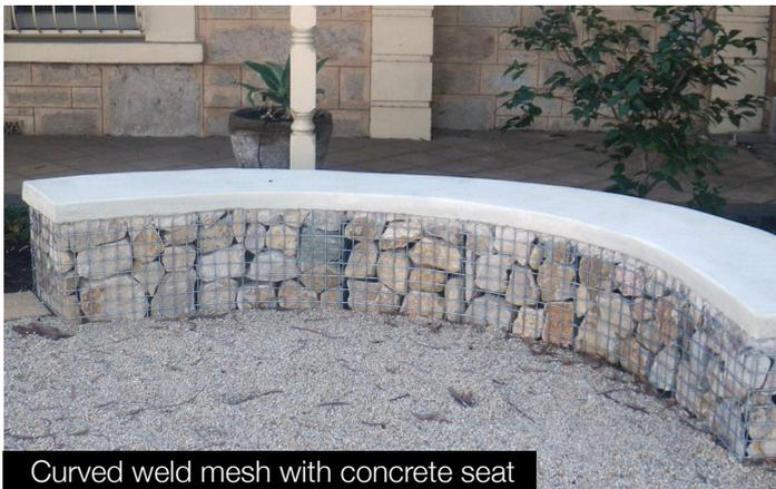
Curved weld mesh with concrete seat
