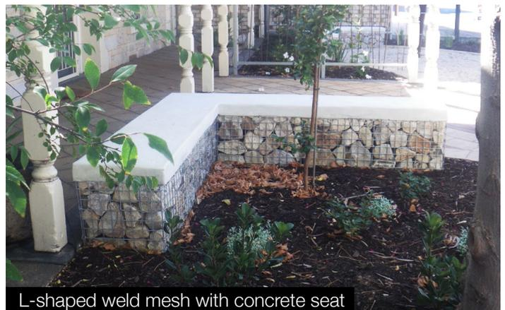
L-shaped weld mesh with concrete seat
